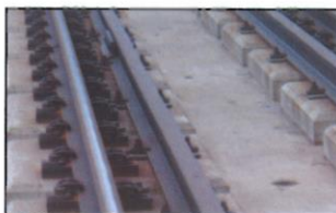
Fig. 3: Short-wave corrugation
