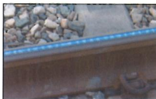
Fig. 2: Short-pitch corrugation
