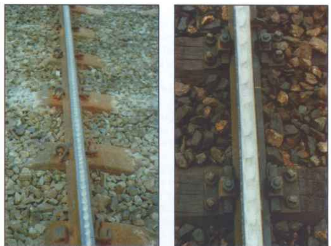
Fig. 1: Short-pitch corrugation (left) and short waves (right)
